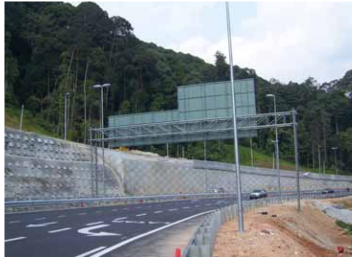
Figure 4: Nehemiah Wall at Ramp
