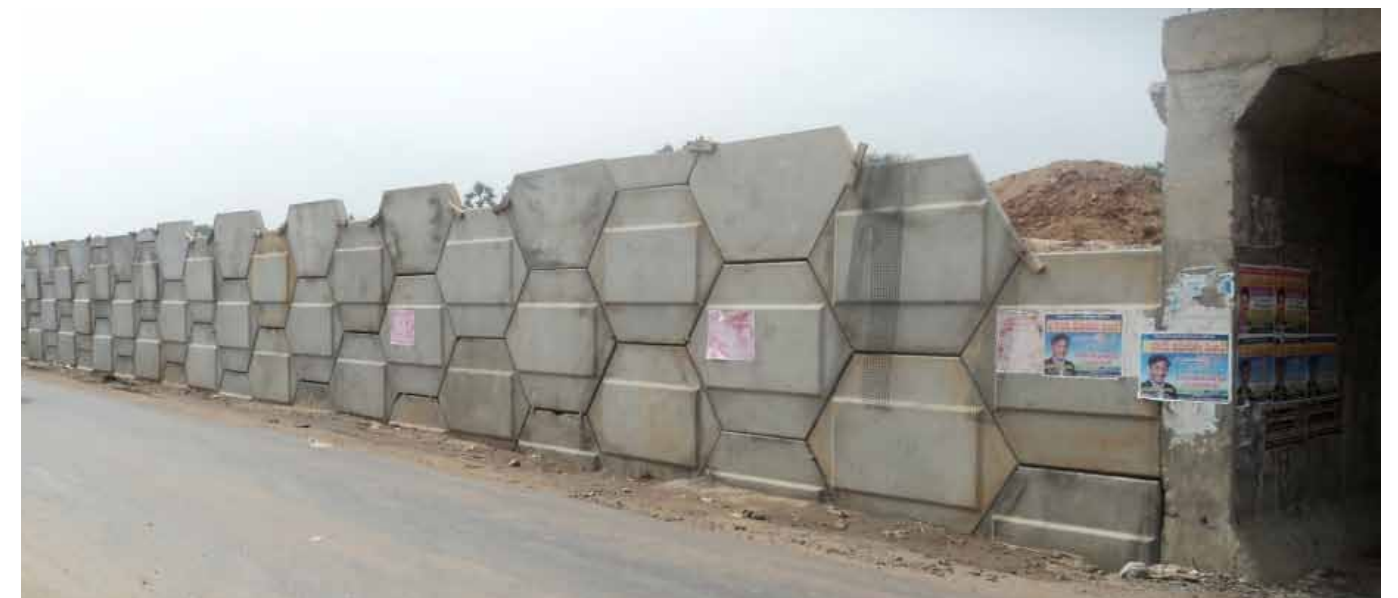
Nehemiah wall at bridge abutment
