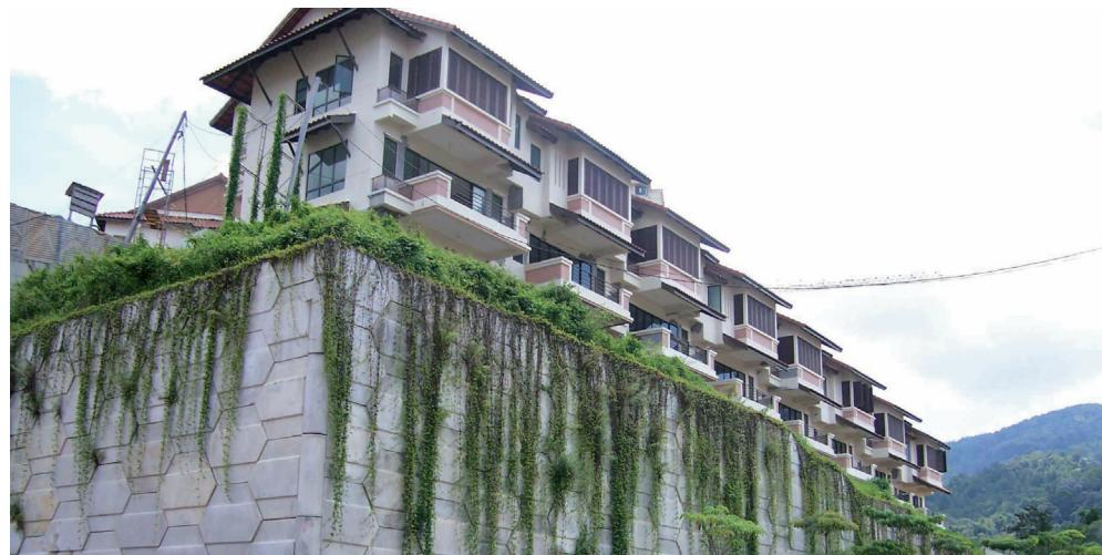
**Rock solid:** The Alila housing project in Penang uses the Nehemiah Wall for slope protection
